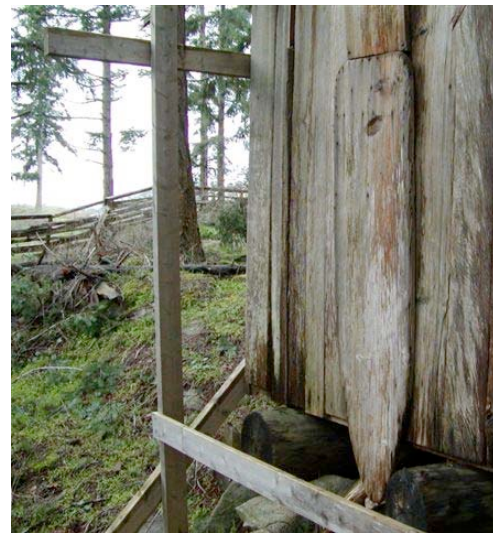
Ironing board used as a patch on the Boatbuilding Shed.
